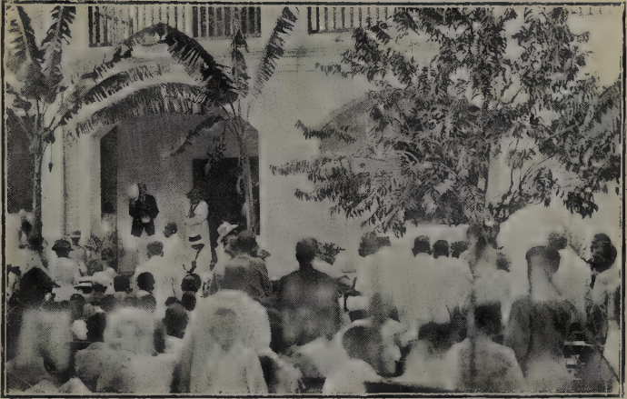
OPENING OF THE CLASSROOM BLOCK 1923
